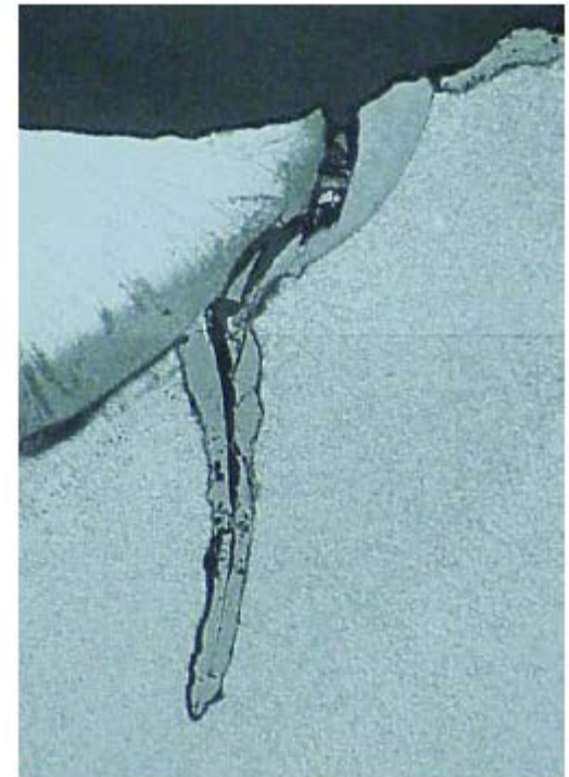
Superheater tube attachment fatigue cracking
